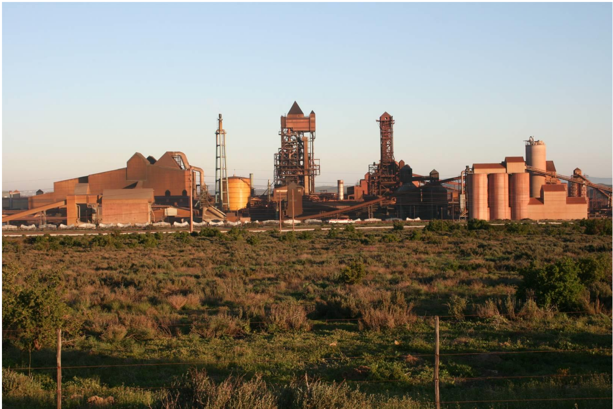
ArcelorMittal South Africa's Saldanha steelworks are ideally suited for green steel production. Image supplied
